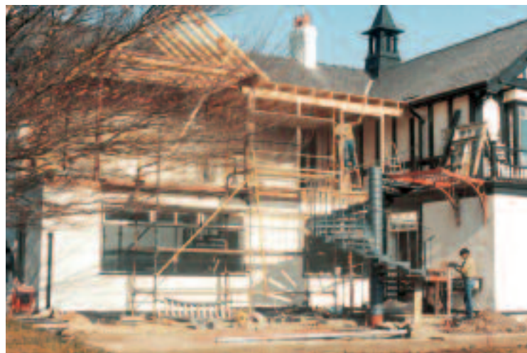
THE EXTENSION BEGINS WITH THE CONSTRUCTION OF THE FIRE ESCAPE
